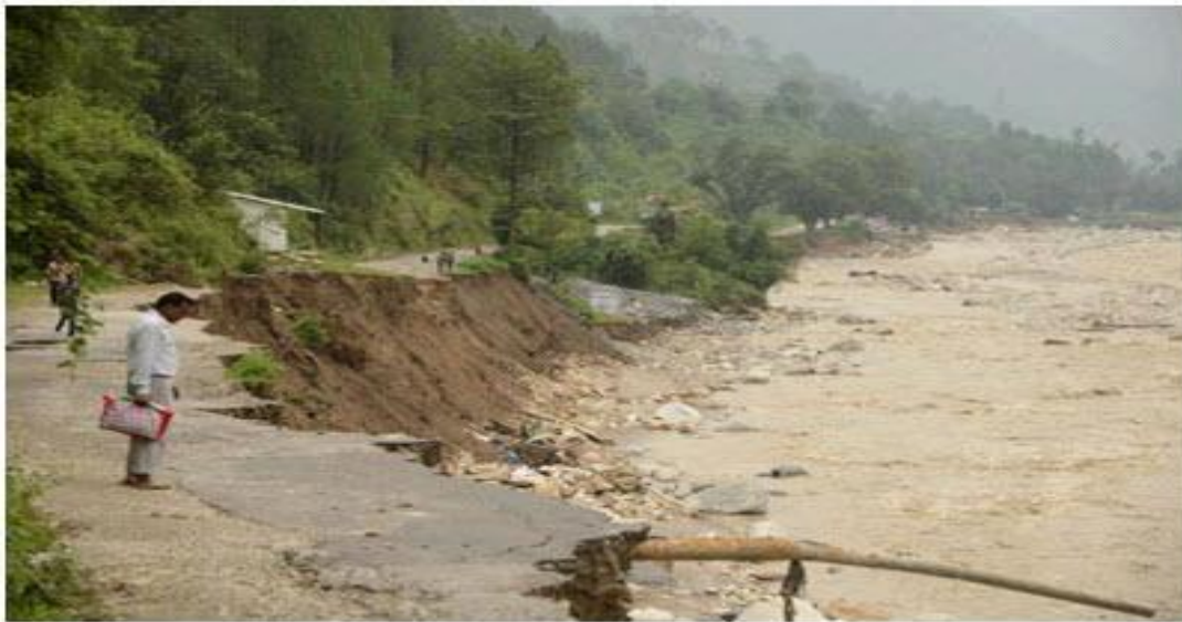
Fig. 1.7 Stream bank erosion in mid Himalayan region of India
